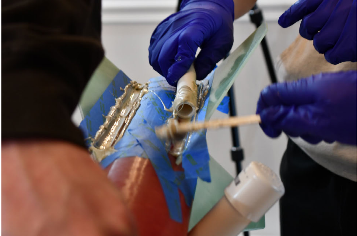
Image 18: Applying external fillets.
